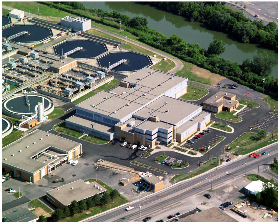
Metropolitan Syracuse Wastewater Treatment Plant
