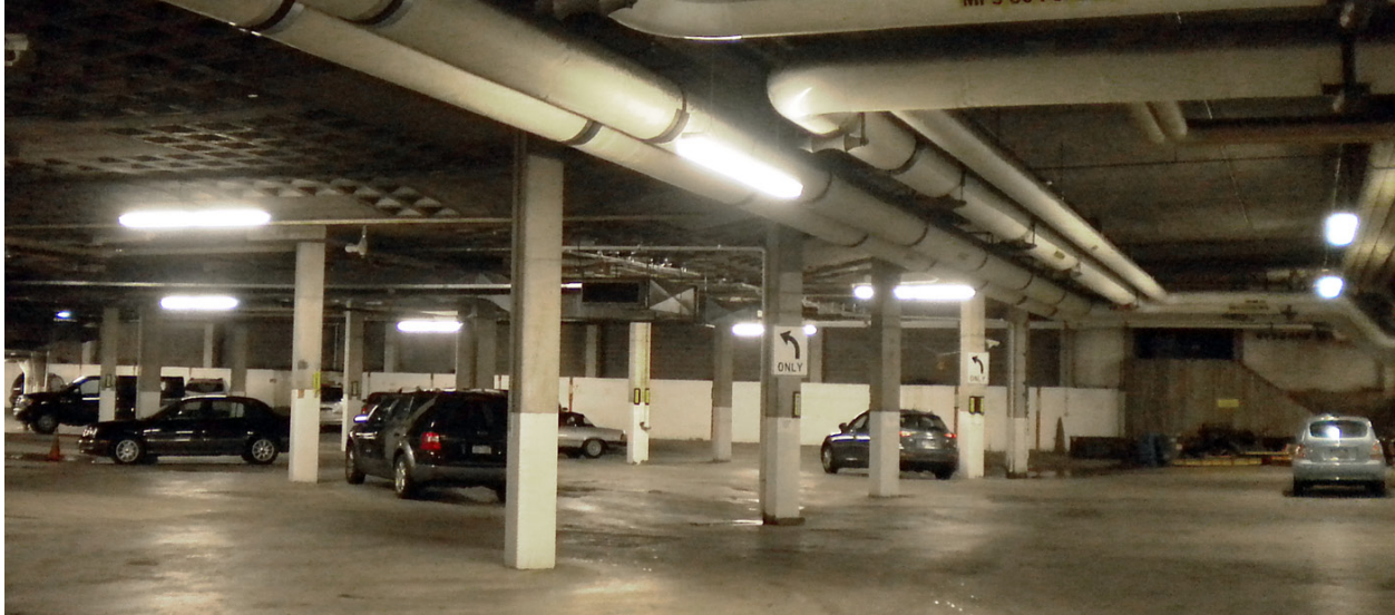
County lighting project
