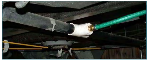
A garden hose creates a dangerous cross connection between potable and non-potable water.
